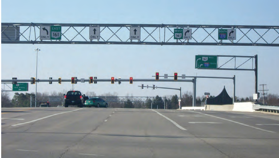
Figure 23. Mast-arm mounted lane-use control signs
