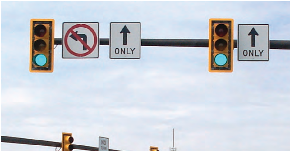
Figure 24. Yellow retroreflective backplates
