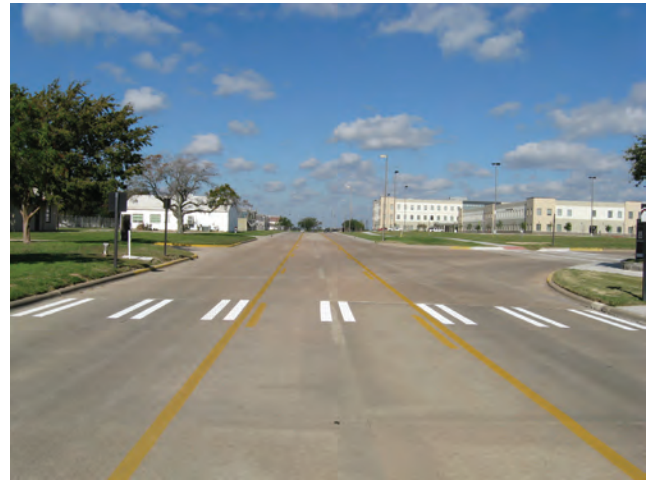
Figure 88. Example of bar pairs crosswalk markings
