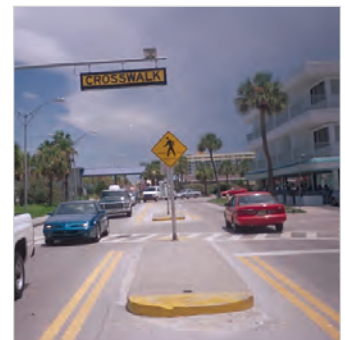
Figure 11. Raised median island with yellow marking on the vertical face and top surface
