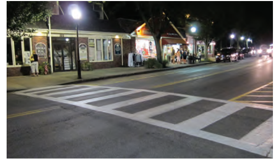
Figure 36. High-Visibility ("Ladder") Crosswalk
