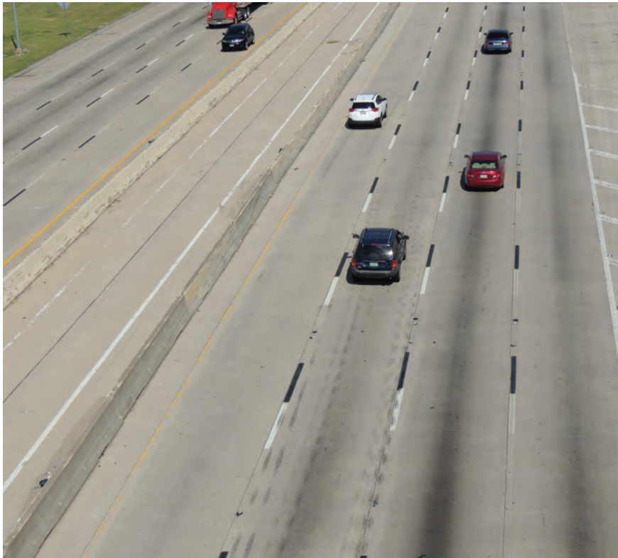
Figure 57. Contrast Markings on Light Colored Pavement
