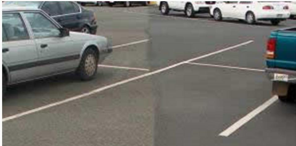
Untreated (left) – Sealed Treated (right)
