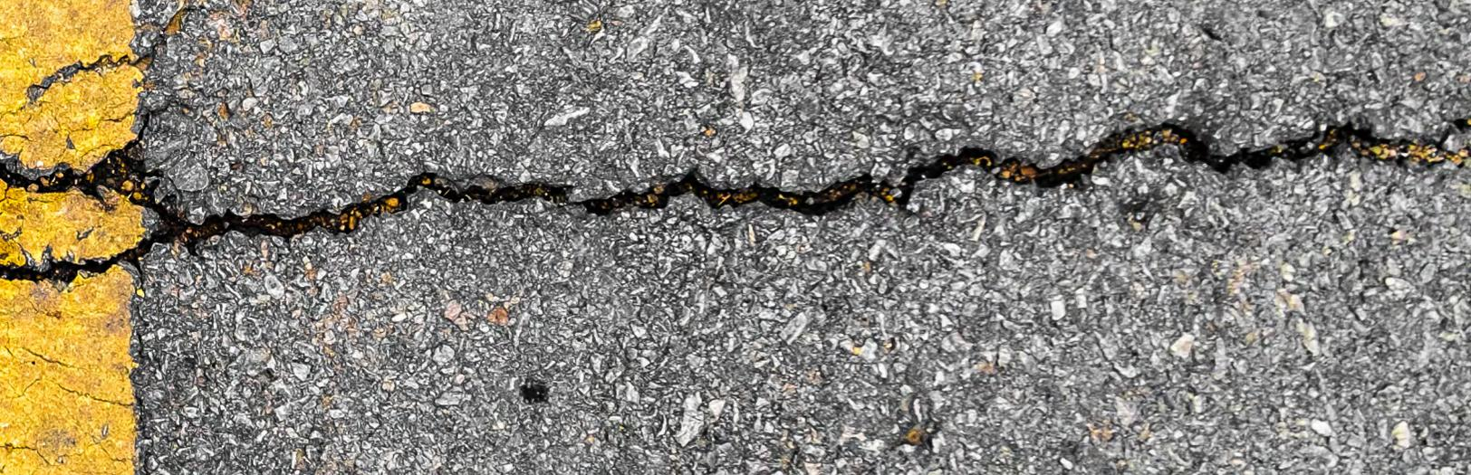
Traffic should not be allowed on the sealed cracks until the sealant has cured. Blotting with an application of fine aggregate can protect the sealant from tracking or prevent the surface from losing friction.
